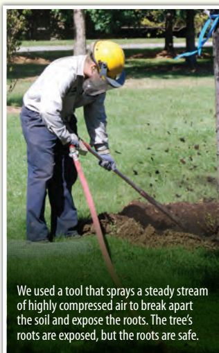
Next, we found one of the larger roots and used the air tool to pull away all of the soil and follow that root to its end. We used a non-toxic spray paint so the tree root could be easily identified.
